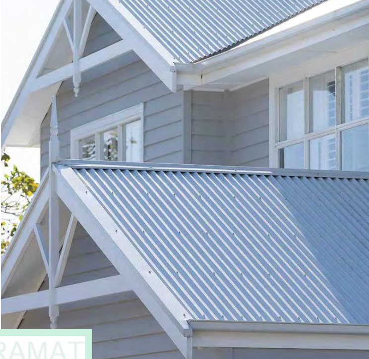
SHEETING TYPE 1 - CUSTOM ORB ACCENT 21 IN SURFMIST PIPES - SURFMIST FINISH TO MATCH RF01 ERS & EAVES - SURFMIST FINISH TO MATCH RF01
