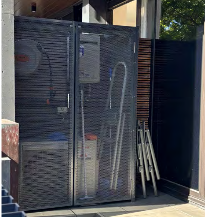
MS01 - MESH SCREEN WITH DOORS POWDERCOATED TO MATCH BRICK COLOUR (MIN. 70% FREE-AIR REQUIRED)
