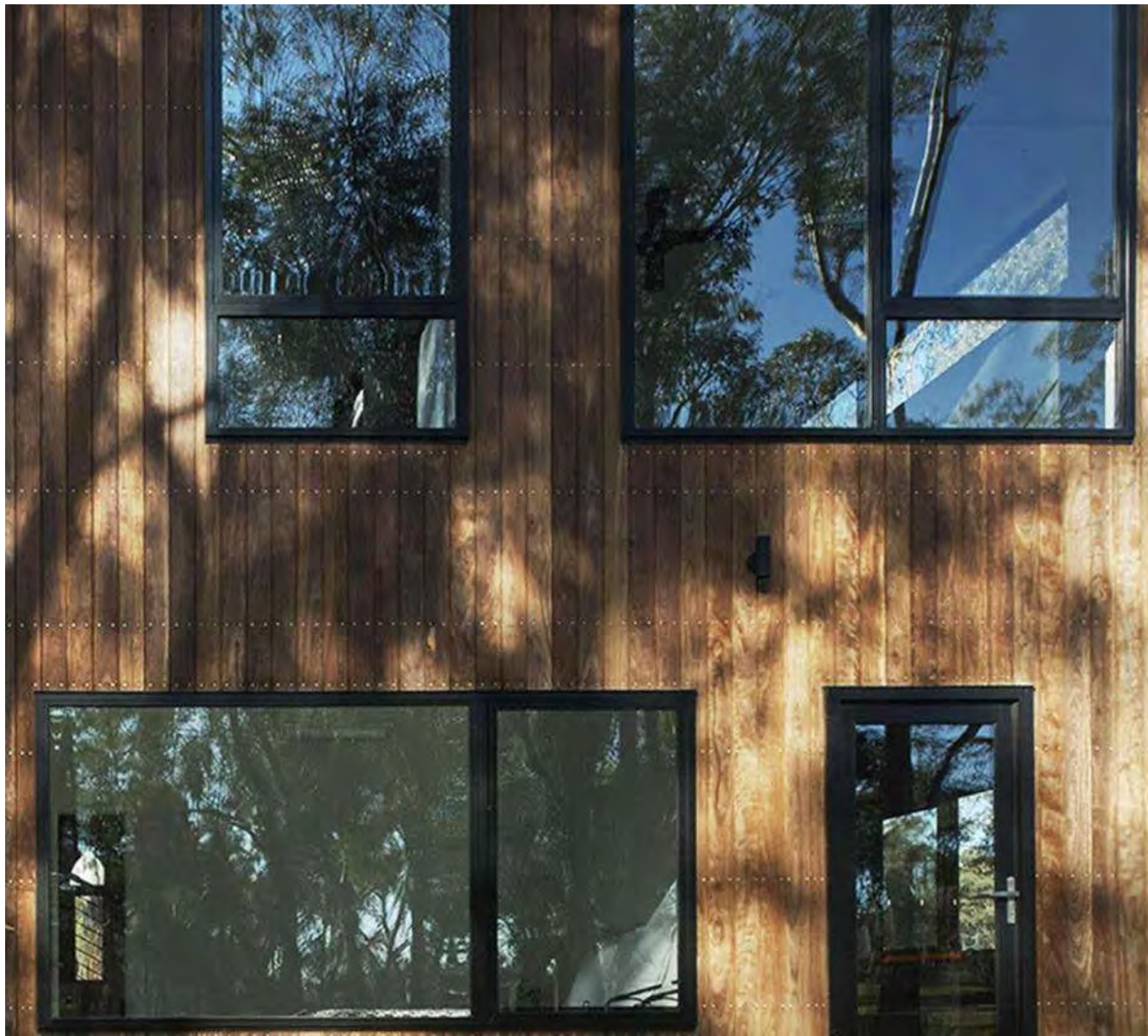
AL01 - ALUMINIUM WINDOW FRAME TYPE 1 - MONUMENT POWDERCOAT
