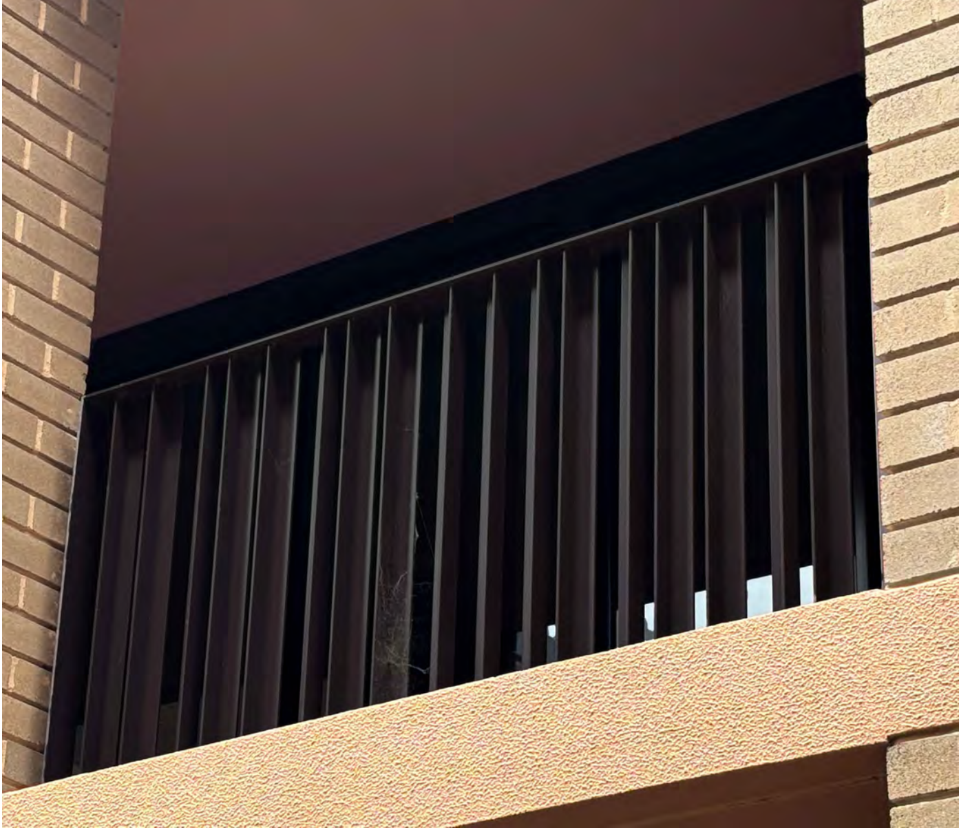
MW01 - METALWORK TYPE 1 - RAILING IN MONUMENT POWDERCOAT FINISH OR EQUAL
