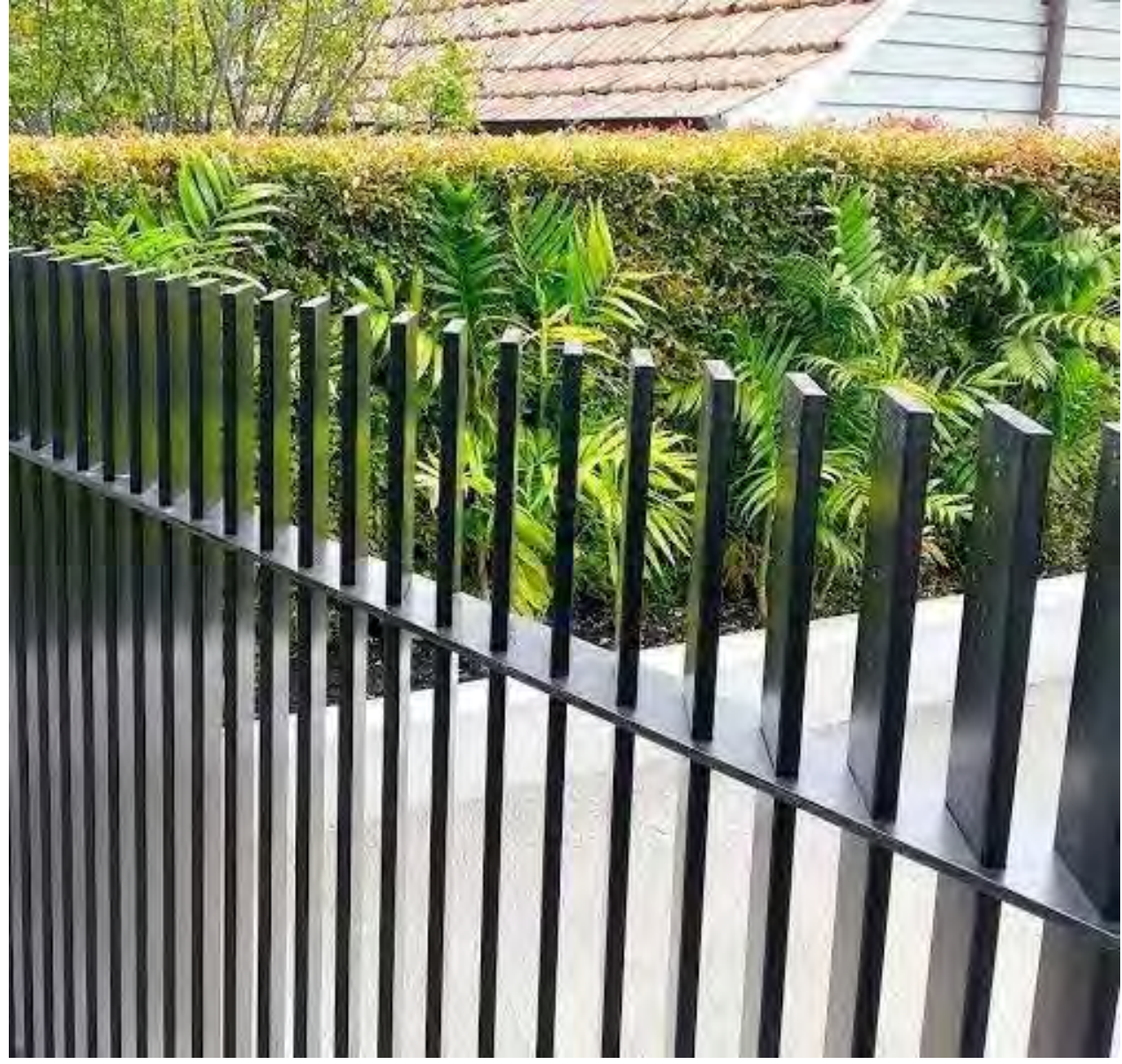
FEN01 - FENCING TYPE 1 - 45° PALISADE MONUMENT POWDERCOAT ON BRICK PLINTH OR EQUAL FEN02 - FENCING TYPE 2 - 45° PALISADE MONUMENT POWDERCOAT OR EQUAL
