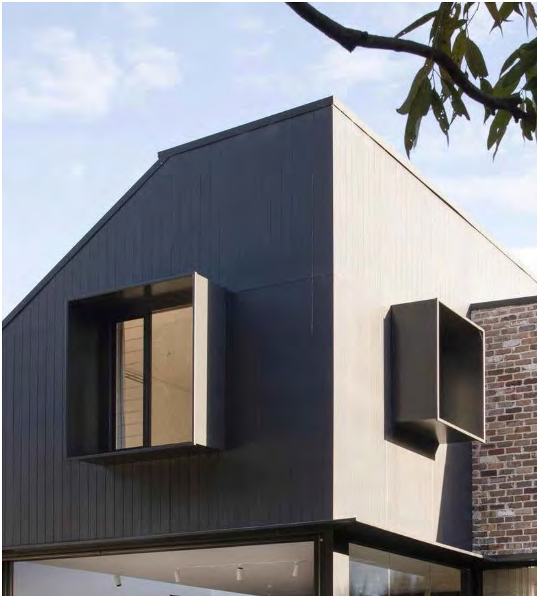
SD01 - SHADING DEVICE TYPE 1 - HEKA FULL SURROUND HOOD IN MONUMENT POWDERCOAT FINISH
